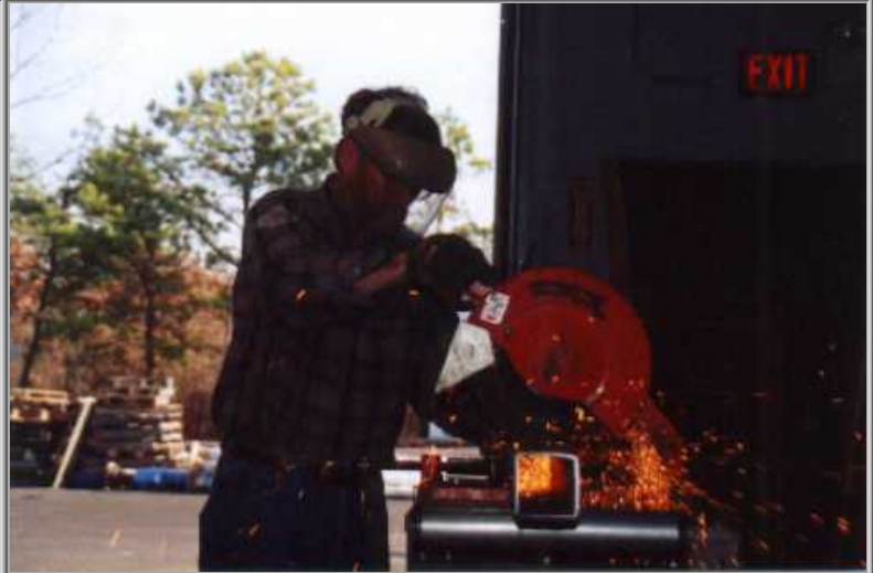
The 3"x3" tube steel is being cut in the correct size pieces and its ends with the correct angles using a chop saw
