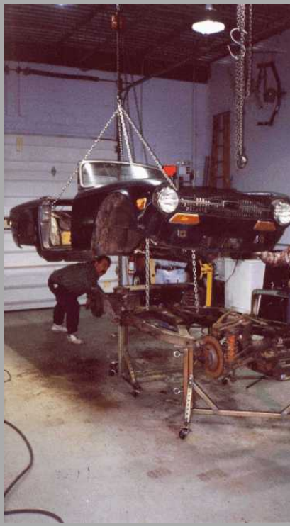
Pyramid chain structure was formed at c/g of body. All body/frame mounting points were removed (18 in total)
